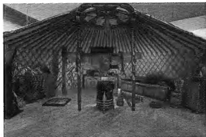
A traditional Mongolian nomad dwelling—called a ger—made of a wood frame and covered in heavy felt.
